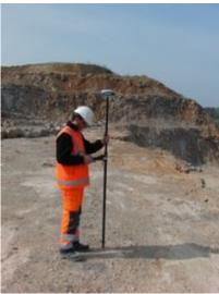
To verify that the drilling matches the implantation, the exact hole position is taken with a precision GPS. Then each hole is checked, using an inclinometer sensor to monitor any possible deviations wich might occur during the drilling.
