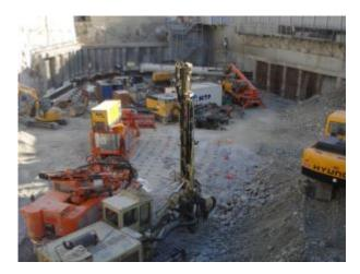
**MICRO-BLASTING** is a technique for clearing rock rubble with explosives. the use of micro-loads between 100 end 2000 grams minimizes the vibrations of the blast impact on the surrounding structures. This techniques results in a significant reduction in daily vibration and noise limitations imposed on the daily use of a hydraulic rock breaker (noise, dust, slow place...).
